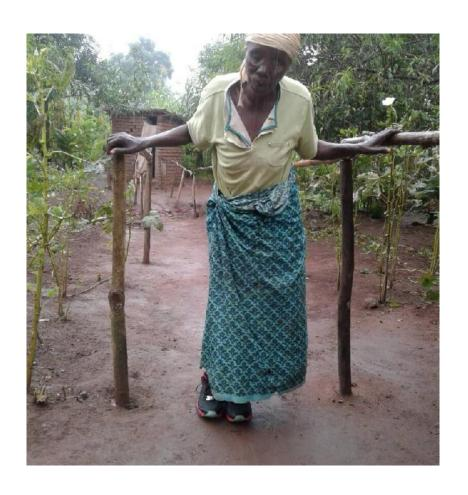
A pit latrine adapted to assist a visually impaired family member with handrails and raised seat inside the latrine.
