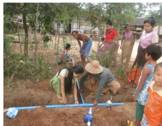
Villagers in Nat Gyi village build a water pipeline connection.
