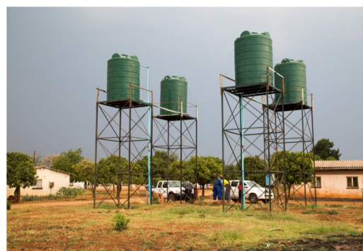
Newly installed Water Tanks for Kadoma City Medium Security Prison
