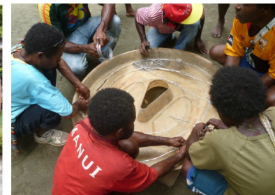
Toilet construction training in Wewak – facilitated by IRDI
