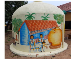
Left: Rainwater harvesting system constructed at Nuffield School for visually and hearing impaired children. Right: The late Elena Down from cbm helping NPCODA and WV on how to raise awareness on disability and the UNCRPD.
