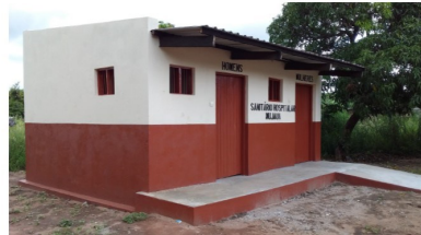
An accessible sanitary block at a health centre in Cuamba.
