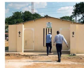
Rehabilitated Public Toilets – Mubaira Growth Point, Chegutu
