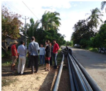
Main pipe installation and water service provider at Sambok commune Chettr Borey district Kratie
