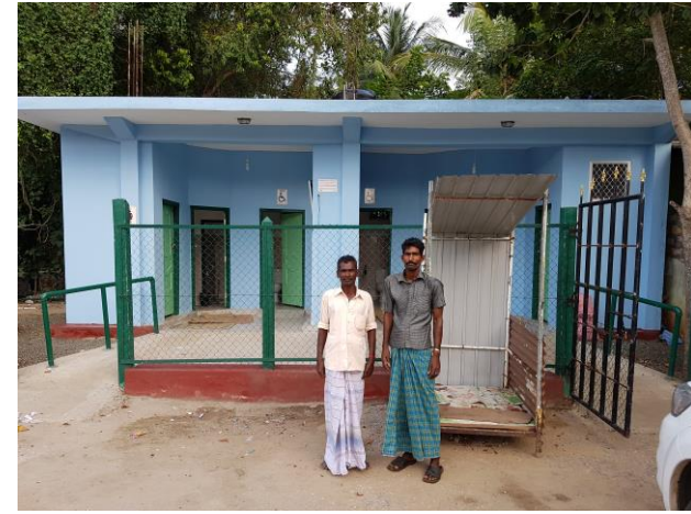
Public toilet with universal access
