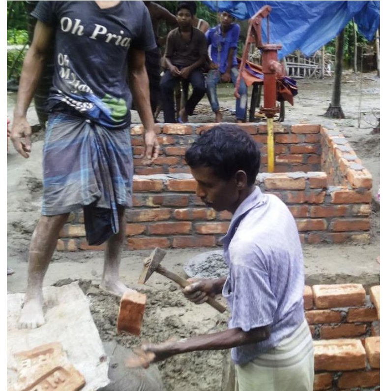
Rehabilitating tube-well platforms to remove the bacterial infection in drinking water
