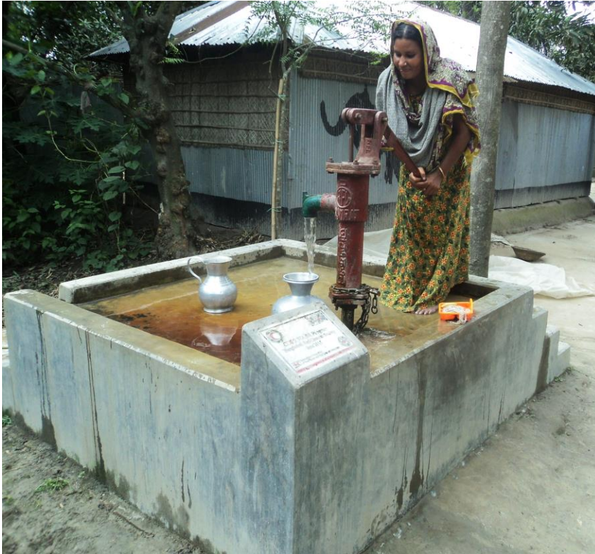
Installation of new tube-wells addressing flood level in Rangpur to increase the sources of drinking water
