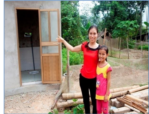
Hygienic latrines just built thanks to WASHOBA project in Thai Nguyen
