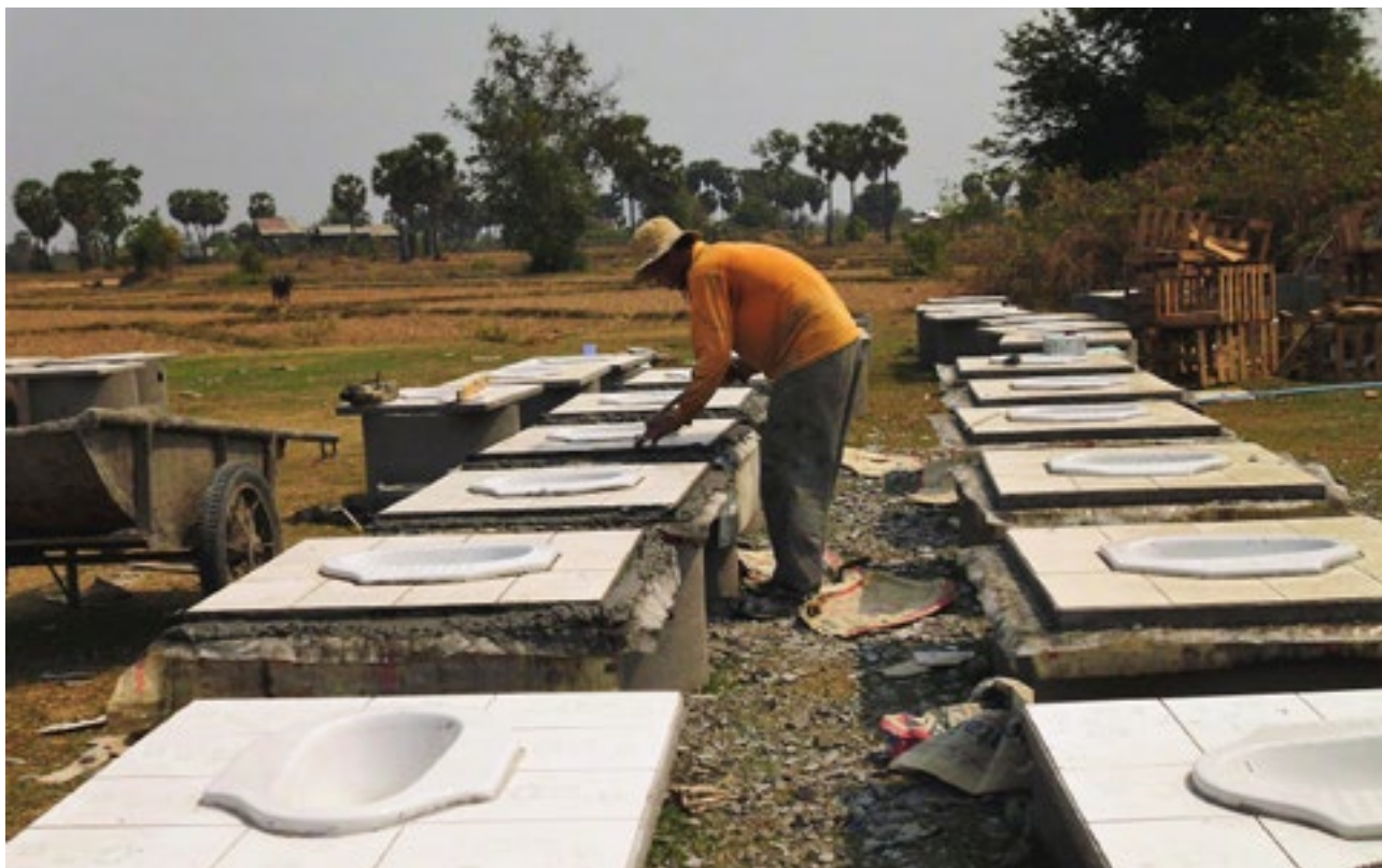
Kampong Cham province on-site latrine component construction. Photo credit: Thrive Networks
