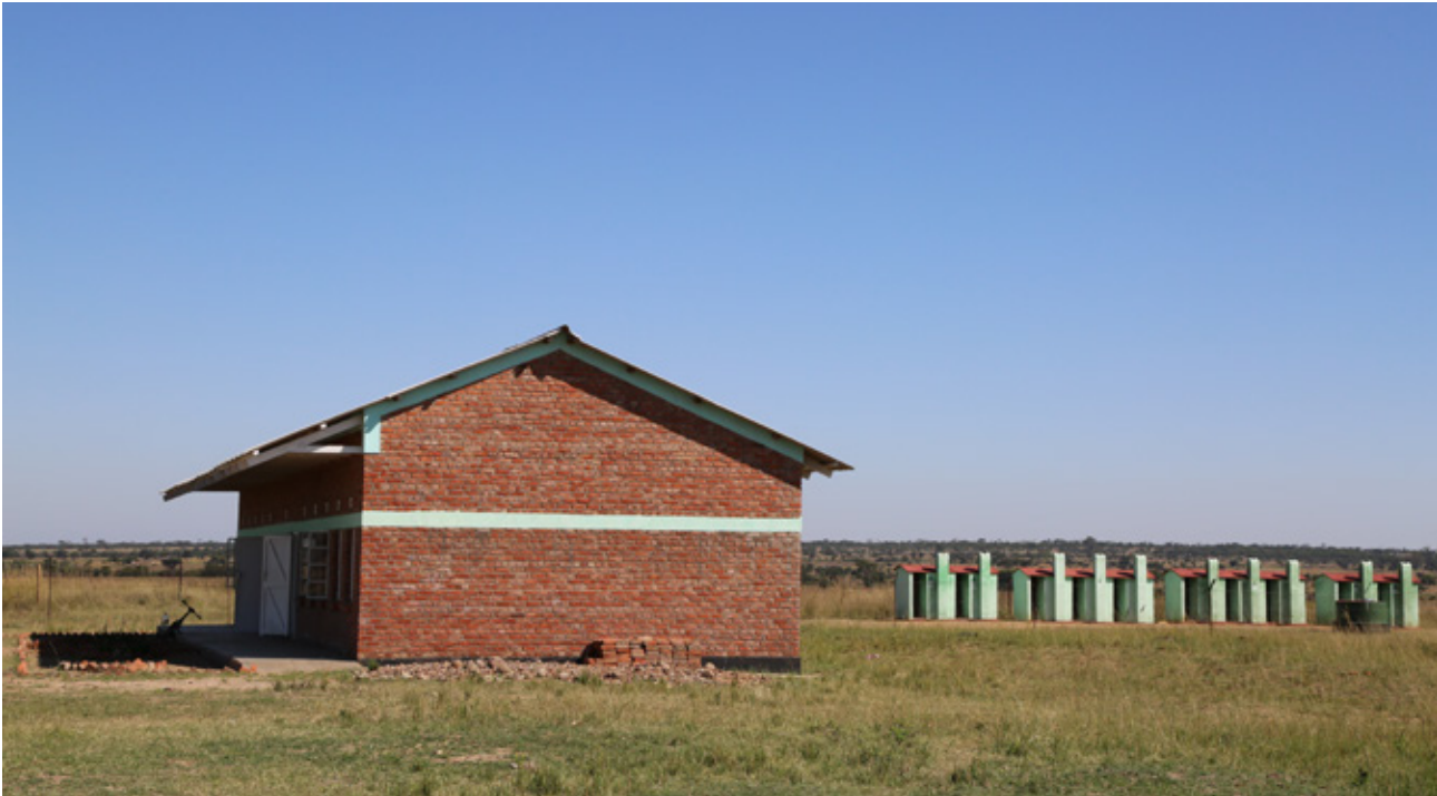
A primary school and toilet blocks in Norton, Zimbabwe.
