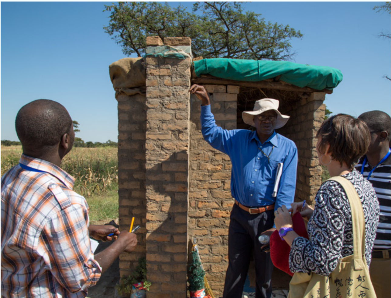
An ungradeable Blair ventilation improved pit latrine.
